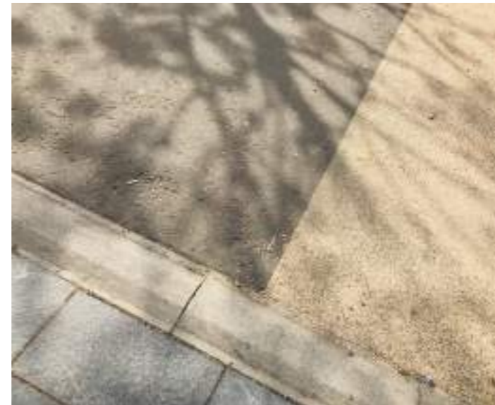
Central delineator strip / for cycle track/footway surface where it is not possible to achieve a total separation between the footway and cycling route for example, at limited pinch points.
