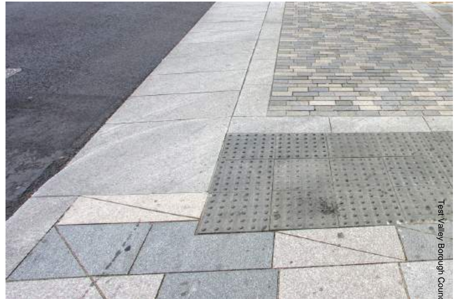
Good side street detailing / Sidcup
