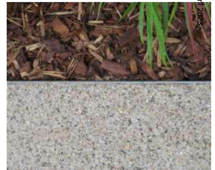
Steel edging / separating resin bound gravel path from planting area.
