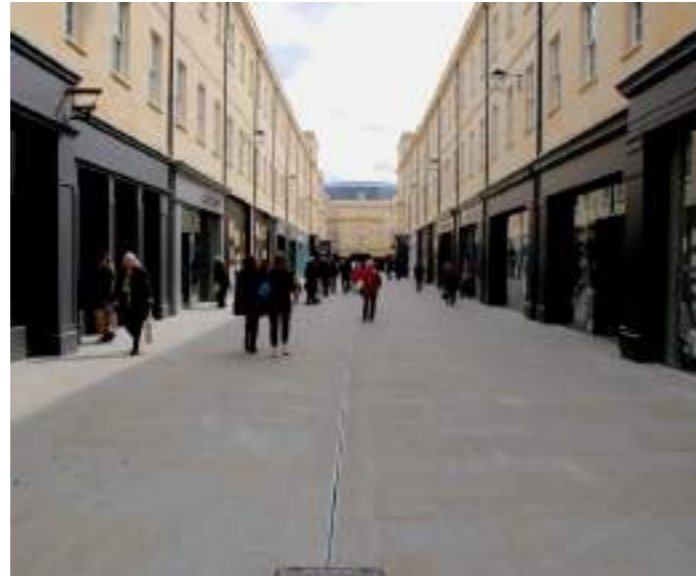
Unobtrusive longitudinal pennant sandstone flag channel / laid flat directing surface water to linear slot drain and gully in the City of Bath
