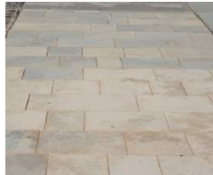
Purbeck Limestone / Flag paving, sawn edge, 400mm wide x random lengths.
