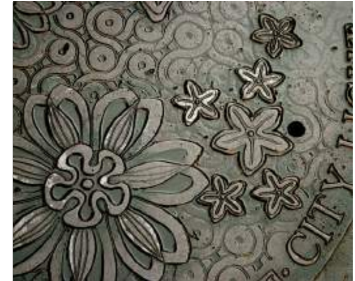
Bespoke cast iron manhole access cover incorporating art / interpretation as shown here in Seattle.
