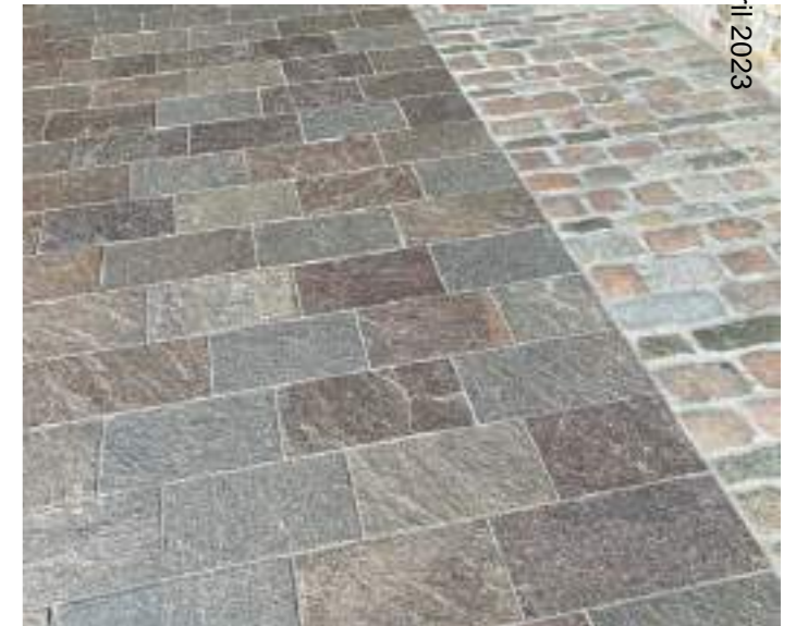
Porphyry flags / meet reclaimed granite setts at a building interface in Coal Drop Yards, London.
