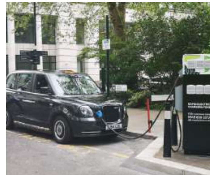
Free-standing rapid charging point / London
