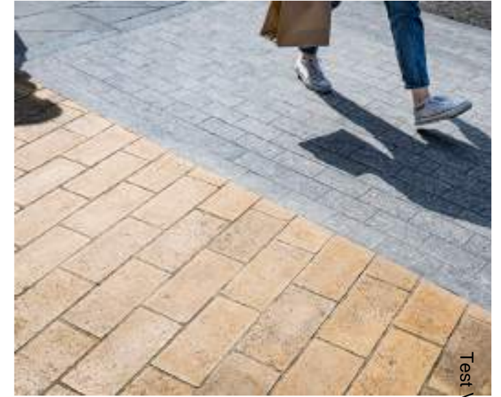
Use of Purbeck limestone setts / to announce a threshold between the high street and a narrow yard as shown along Borough High Street, London.
