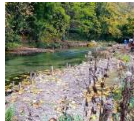
Stabilised channel (establishment)
