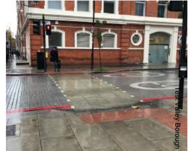
Concrete imprint / used at crossing to harmonise with general footway materials in the street on Camden Road, London.
