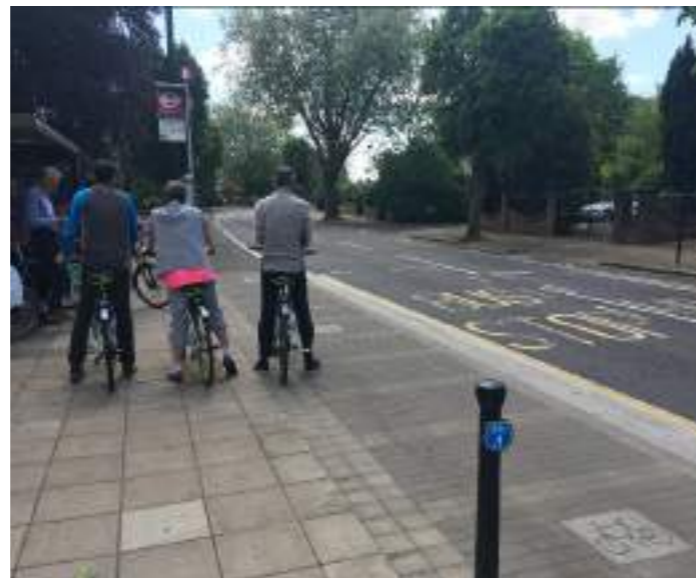
Block Paving / Used here on a bus border as a clear differentiation between footway and cycle track is made.
