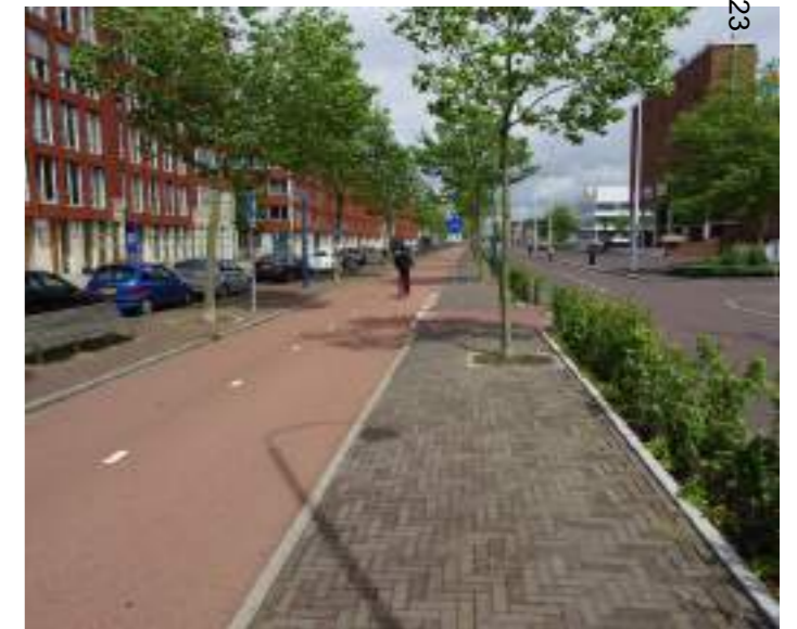
Coloured Asphalt Cycleway and Clay Paver Footway / Monolithic poured material with clay pavers.
