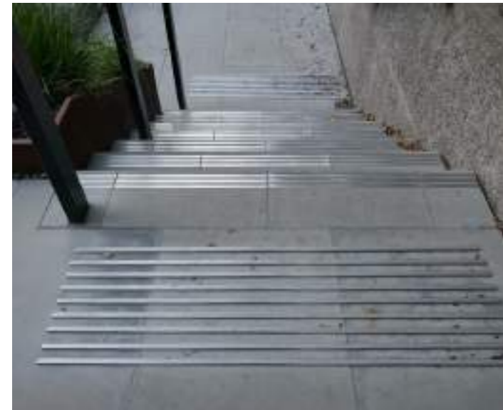
Tactile hazard warning (corduroy) paving / helps visually impaired people anticipate specific hazards e.g. top and bottom of steps; transitions between footways and areas shared with other users as seen here in Salters Garden London.
