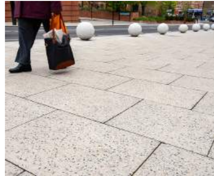
Footway / Enhanced precast concrete flag paving as typical street paving material outside of the Conservation Area.
